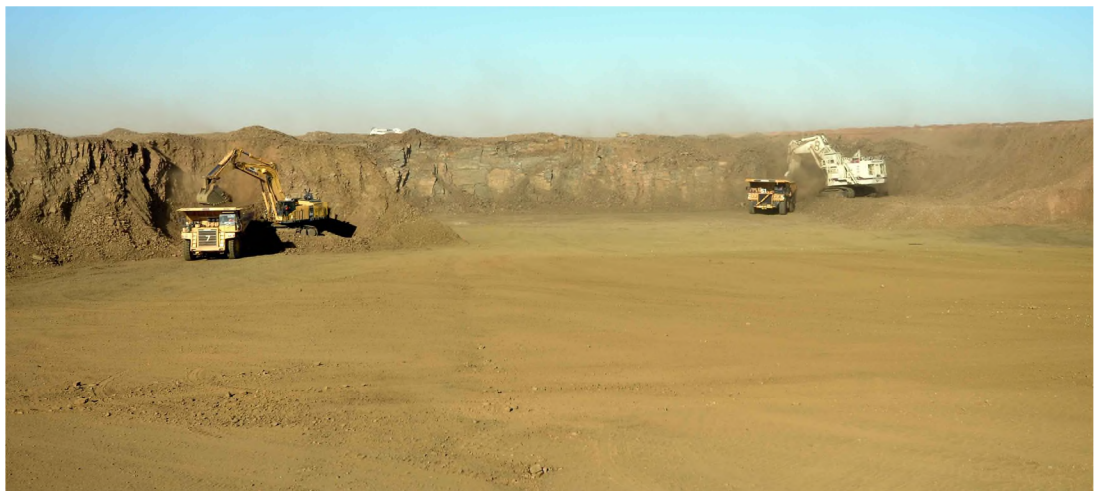
Figure 16-1: Excavators and Haul Trucks Working in West Branch Pit
