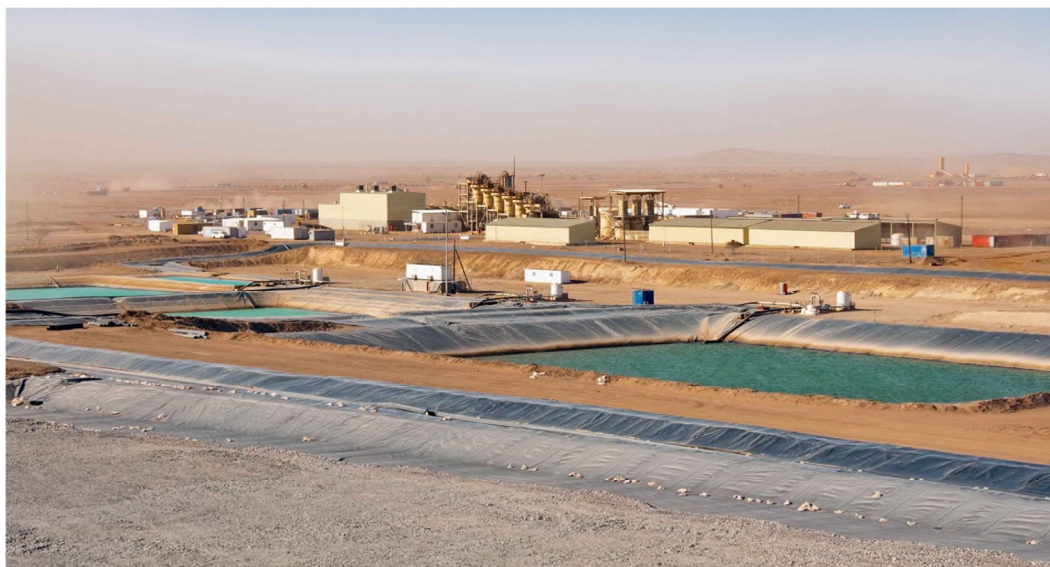
Figure 17-2: West Branch Solution Ponds and ADR Plant
