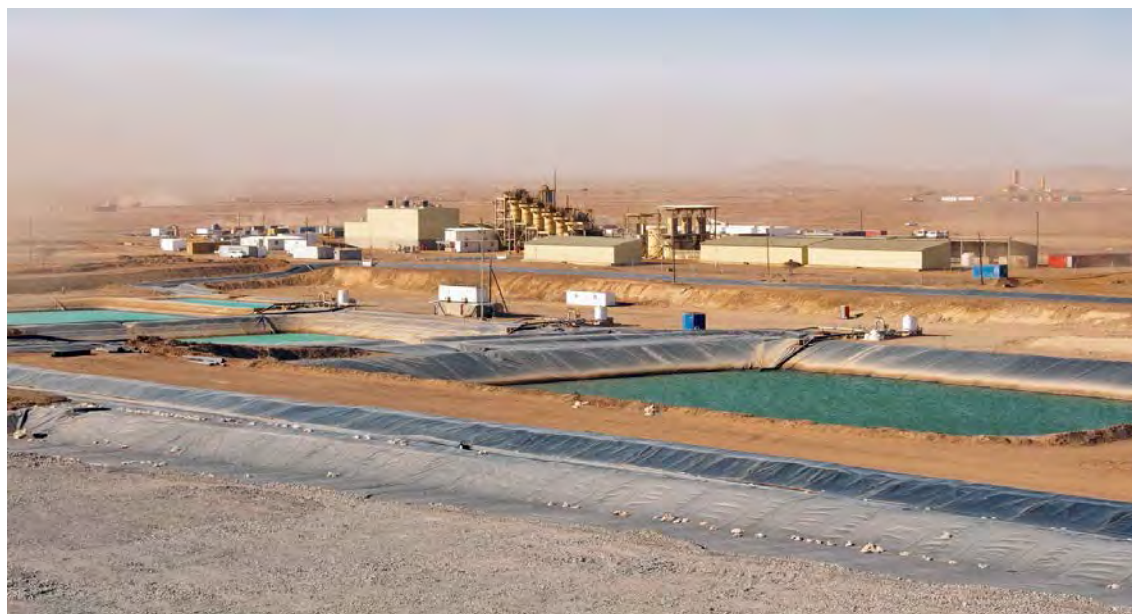
Figure 17-2: West Branch Solution Ponds and ADR Plant
