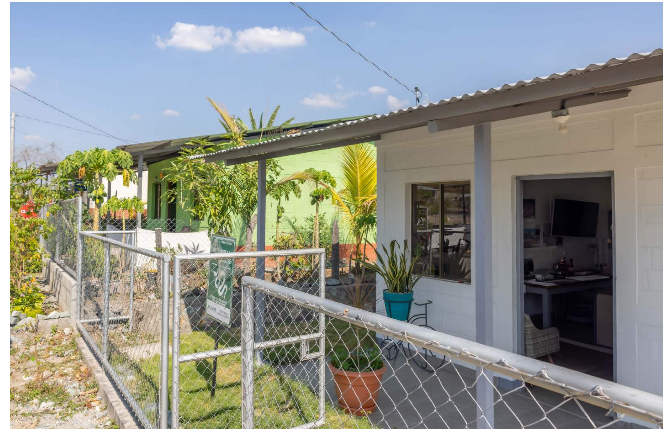
San Gil Resettlement Project, El Limon Complex.
