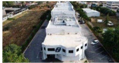
New Athens facility 4,800 sqm
