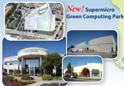
Worldwide Headquarters Campus Silicon Valley, U.S.A.
