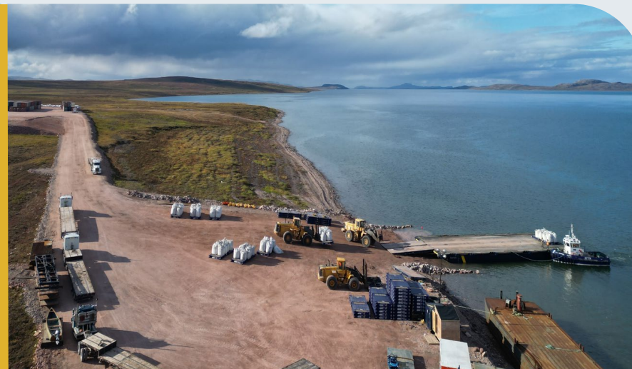
Marine Laydown Area
