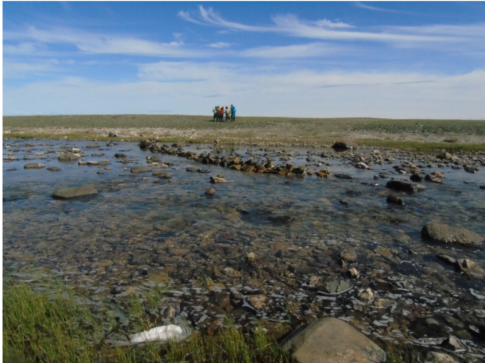
Plate 7.4-2. Directional Weir (Kugluktuk HTO Students in Background) for Migrating Arctic Char in Nulahugyuk Creek, June 24, 2015
