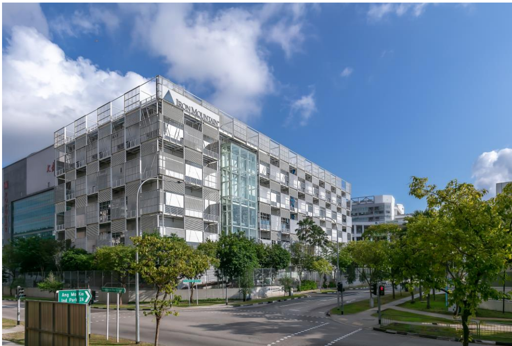
Singapore (SIN-1) Data Center
