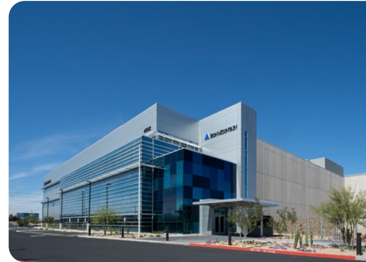
Our Arizona facility AZP2 was the first in North America to achieve the BREEAM sustainability standard. From now on, all of our new data centers will be BREEAM accredited.
